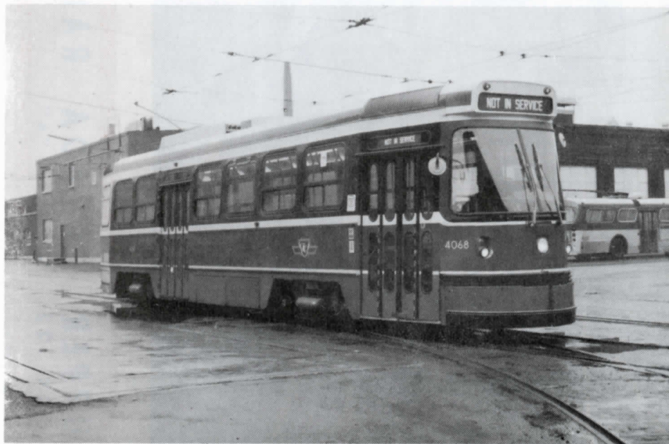
TTC CLRV 4068 is pictured at Hillcrest Shops equipped with the experimental safety covering over the front coupler opening that has been installed on 26 of these cars. The covering may be removed on the street for coupler access.
