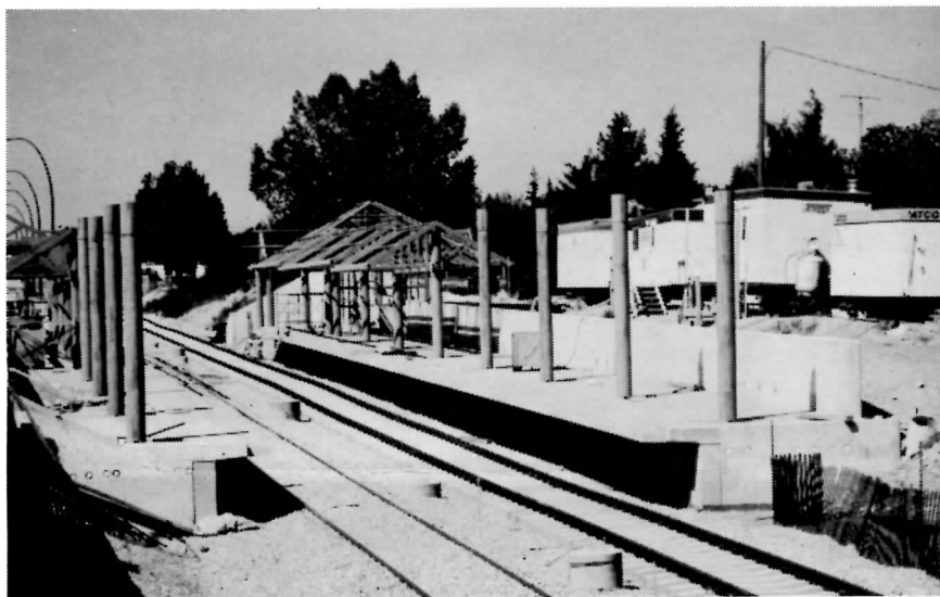
The simple design of the stations on Calgary's Northwest LRT line is evident in this photo. Note the concrete ties. Opening of the line was scheduled for September, 1987. --M.F. Jones
