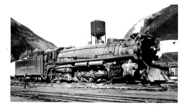
The T-l-a's were the largest locomotives in point of size and weight ever constructed in Canada; total weight of engine and tender in working order was just 375 tons. Their tractive effort was second only to Canadian National's 1924-built 4100-series 2-10-2's, which had a rating of 80,000 pounds.
