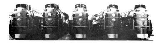
An unfortunate feature of the steam locomotive was that the smoke frequently tended to blow down about the cab, obscuring the engineman's vision, particularly when the engine was drifting. It was this problem which led to the distinctive design of CN's streamlined U-4 4-8-4's.
