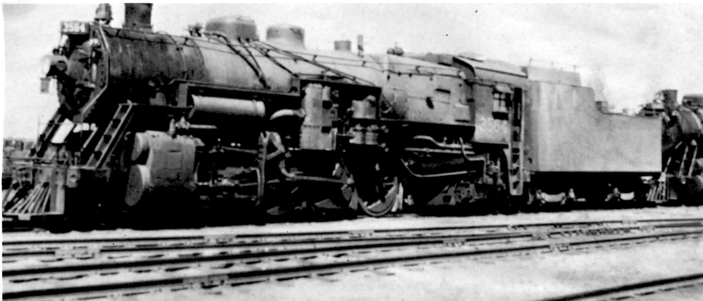
ABOVE - Mikado #3564 was a member of class S-2-b from leaving CLC in 1923 to scrapping late in 1961. Starting out life as coal burners, they were converted to oil in 1953-54. 3564 is shown here in Winnipeg in July 1947. (UCRS coll.)
