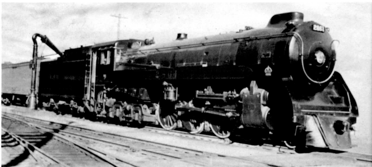
ABOVE BCR Royal Hudson's sister #2861 is seen here taking water. The H1e class engine was built by MLW in 1940. The H1e class (2860-2864) were the last of the Royal Hudsons to be built. (UCRS coll.)
