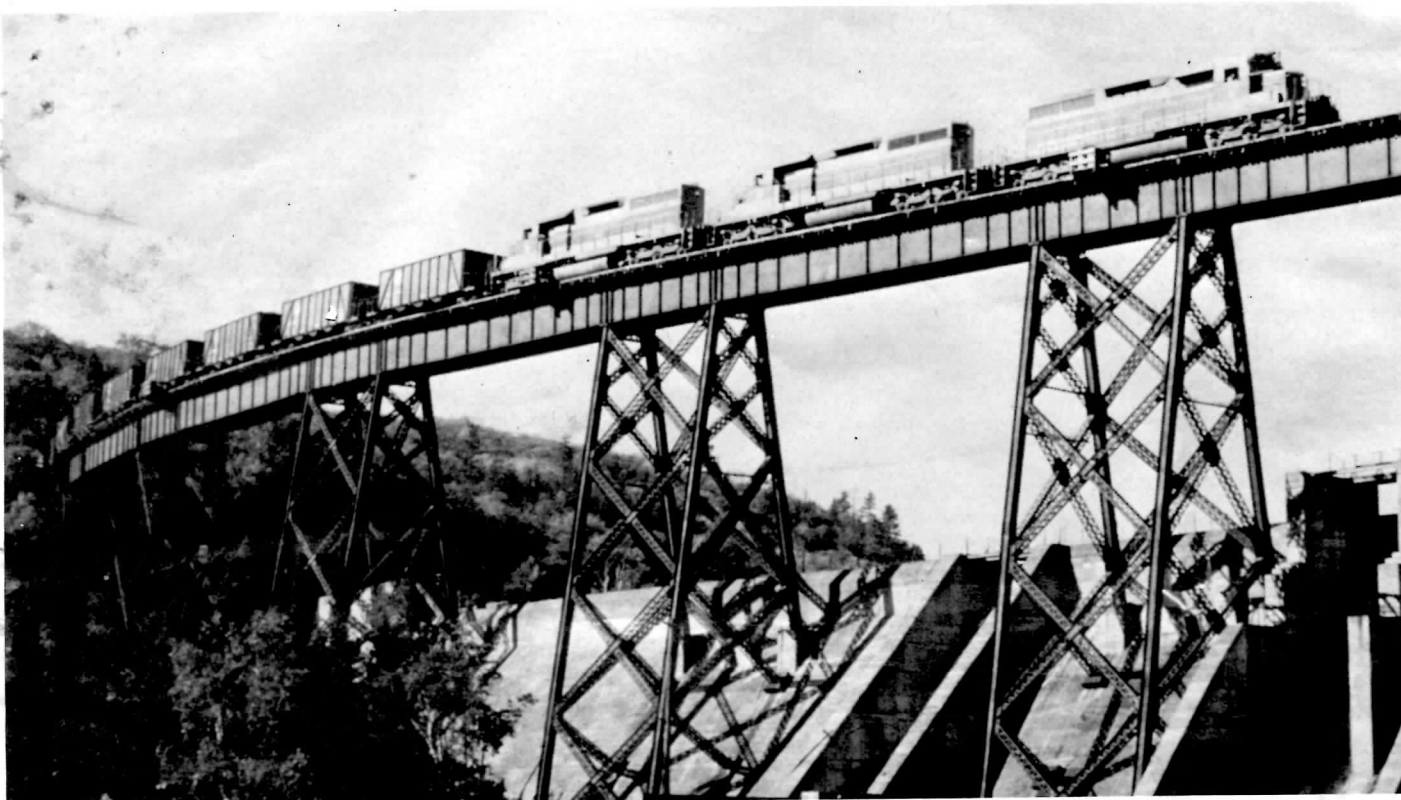
ABOVE - Iron ore is a staple freight for the Algoma Central. A unit train is seen here southbound at the Montreal River trestle hauled by three SD-40's. #180 leads 183 and 182. The low angle of this shot shows how the bridge is built on the side of a Hydro dam. (G. Zuters)
