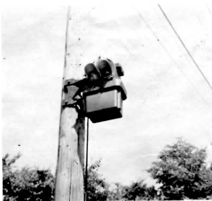
The sidings on the North Yonge Railways were protected by these Nachod block signals, which were activated by a contactor on the overhead which was tripped by the trolley pole as the car approached the siding (J. Bost)
