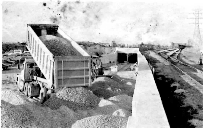
ABOVE: Construction continues on the Eastern Extension of the Bloor-Danforth Subway. Here a truck dumps another load of gravel. Note that the concrete work is complete and the tunnel bore in the rear. 9 Nov 78 T. Wickson.
