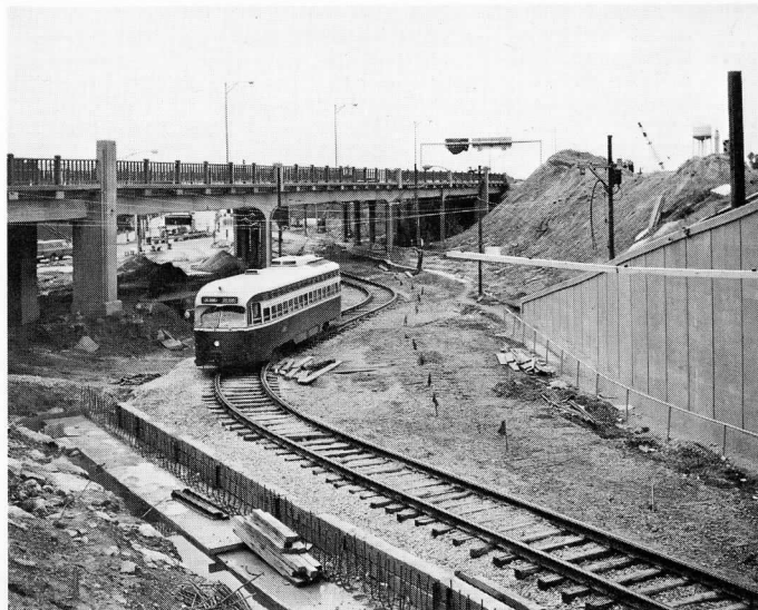
ABOVE: The construction scene looked like this on November 4, 1973 as PCC car #4574 passed through. In the foreground, steel re-inforcing rods are visible. This is where the concrete was poured for the new wall.
