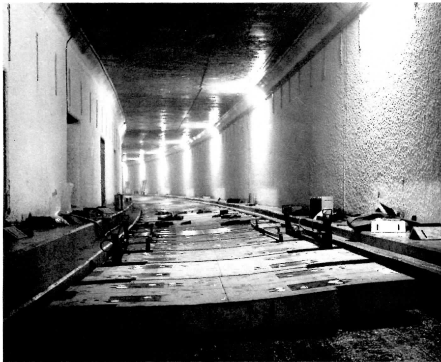
This view of a cut-and-cover tunnel section north of St. Clair West Stn., looking north - west, clearly shows the new railbed arrangement. These double width concrete ties are placed on rubber pads ontop of the recessed floor. The rubber pads are intended to minimise noise. (TTC)
