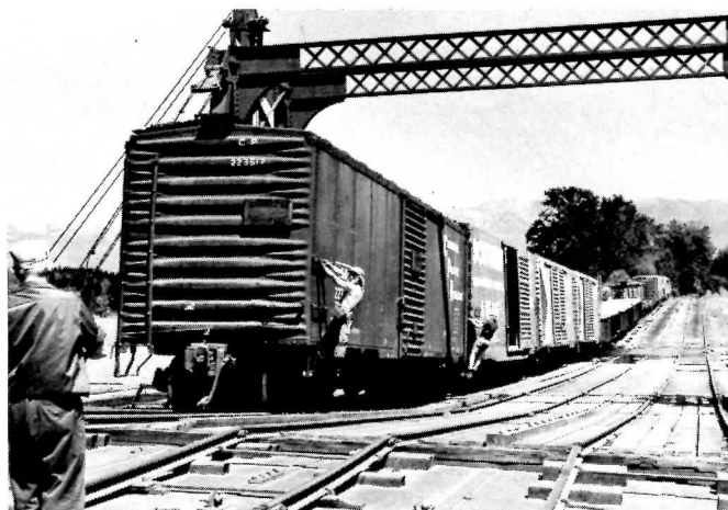
Loading operation at the Proctor B.C. barge slip, with the crew of No. 90 hanging on. Note that the tracks are covered with 3" of water from Kootenay Lake. (KAG)
