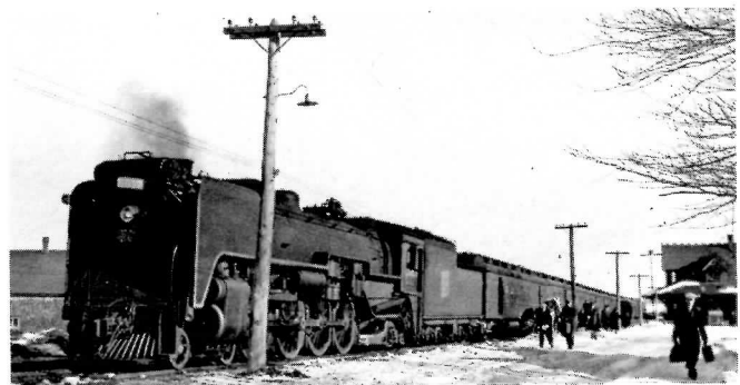
Canadian National 4-8-2 Mountain type 6017 on the head end of what appears to be a local mail and express train. In contrast to the U-1-f class, the U-1-b's did not have the conical bullet nose.
