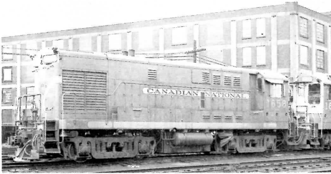
1658-59 were built by CLC in 1956 model H12-44. Shown at Turcot Yard, they were withdrawn from service and retired in December 1968 (D.W.Smith Coll.)
