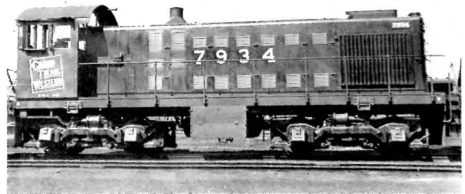
GTW 7800 was built in April 1938 by the Electro-Motive Corporation model SC., was renumbered to 78 in 1950. Powered by a Winton engine, it was retired in April 1962, but was not cut up until 1967.
