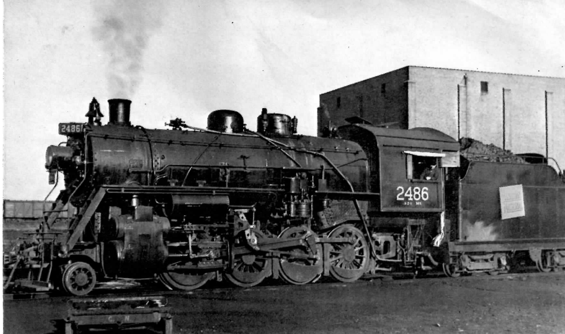
Canadian National 2486 was built by Montreal Locomotive Works in 1918 as Canadian Northern 2486. The N-2-b was scrapped in June 1961.
