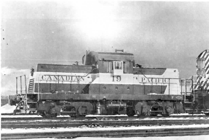
CLC-built diesel-hydraulic switcher 19, shown standing at Agincourt Yard on December 4, has been sold by CP Rail to Penvidic Contracting Ltd. of Burlington, Ontario. The side rods on the unit were taken off for shipment. (Robbin Rekiel)
