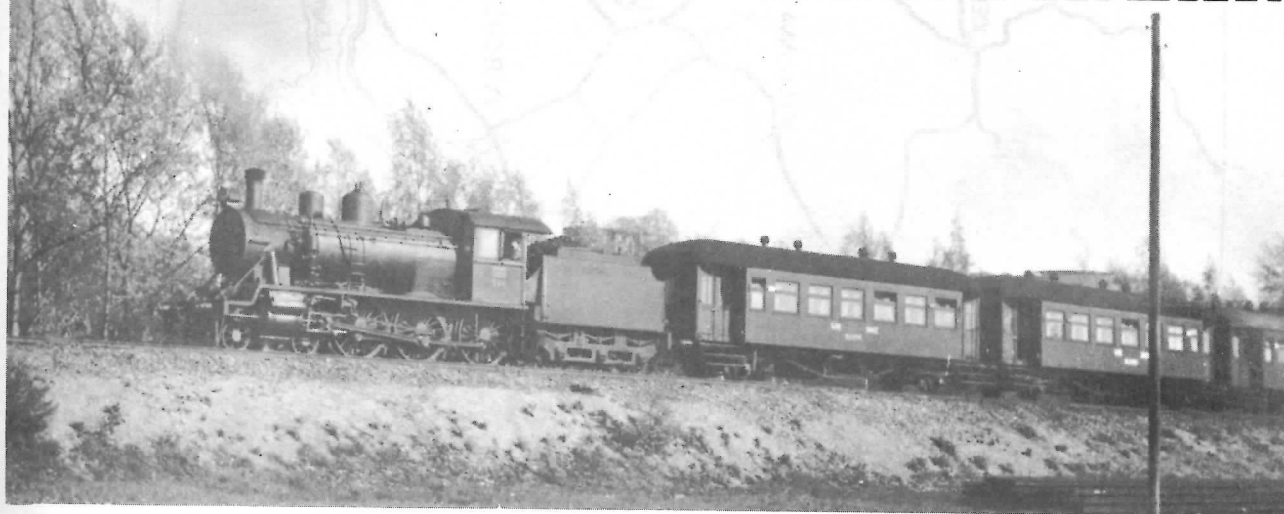
At Pasila engine shed, near Helsinki, no. 586 was seen heading a train of 4-wheeled passenger cars. The engine was built in 1919 by Schwartzkopff of Berlin.
