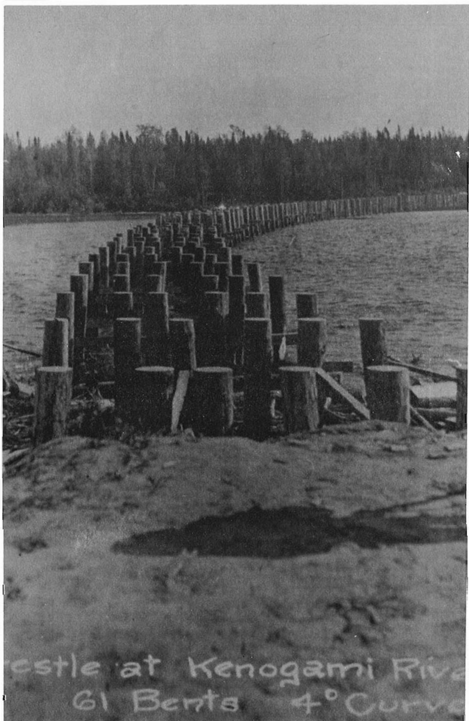
Pilings for the trestle over the Kenogami River at Long Lac, Ontario, the trestle was built on a 4 degree curve and required 61 'bents'.
