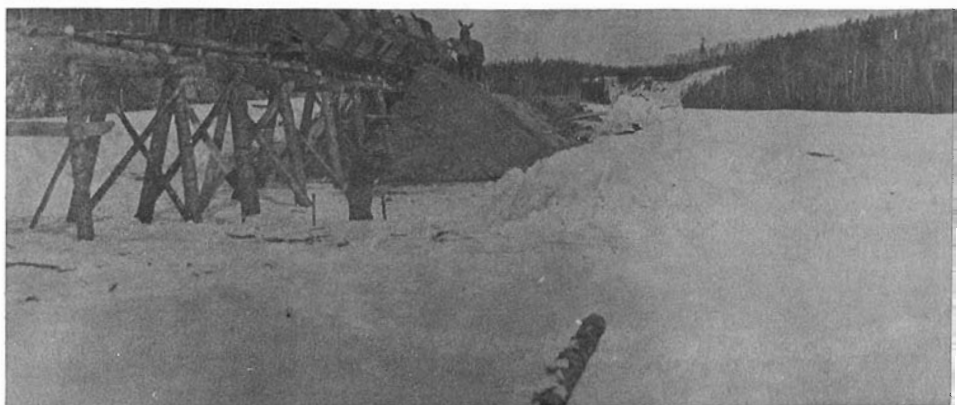
Animal power pulling narrow gauge lorries was the order of the day as workmen dug through this clay cut at mile 86, the lorries were transferred to locations requiring fill as noted in the second photo. View of yet another extensive cut under construction near the town of Nipigon.
