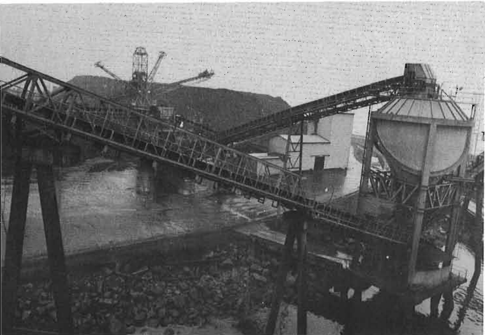
Assortment of conveyor systems within the stockpiling area. Coal arriving from a unit train can be distributed to any one of four stockpiling areas, or directly to the shiploading system. Hopper and delivery systems are flexible and allow changes in stockpiling requirements.
