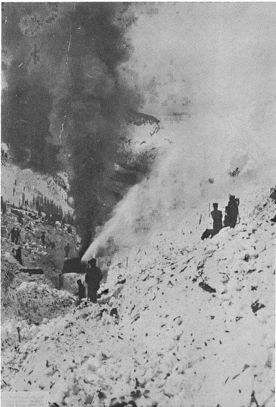
THE ROTARY IN ACTION WAS A SPECTACULAR SIGHT as can be seen from this photo taken in 1910. The scene is probably Rogers Pass after a disastrous snow slide. Pieces of broken trees mixed with the snow were always a hazard to operation of rotary plows.
