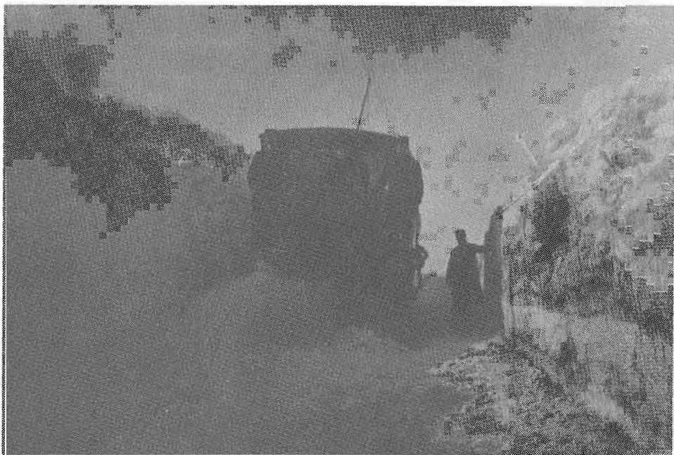
ON DAVIDSON STREET ON FEB 20 1904, a sweeper clears snow from a cutting which was previously cut through by a rotary plow. The snow is almost as high as the car. C.R.H.A. Archives.
