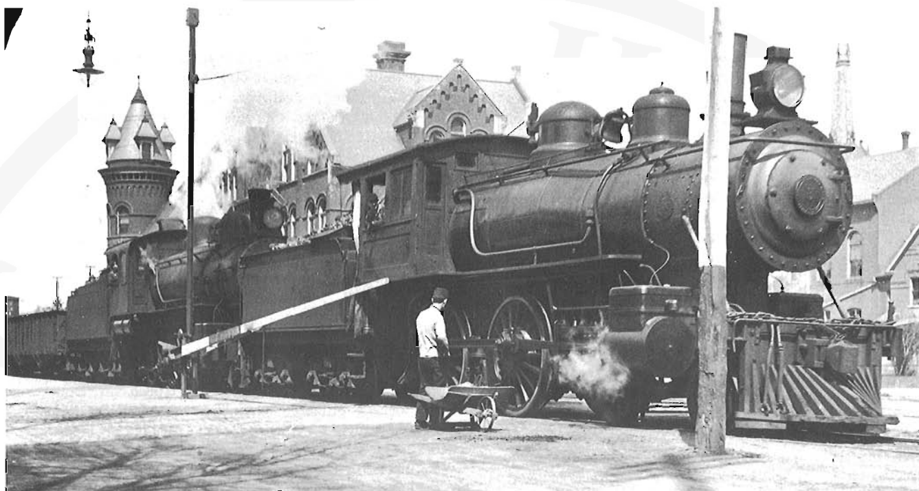
Hauling a freight train, engines 5 and 30 pause at the Hunter Street station in Hamilton in this 1911 view. This is the second locomotive to bear the number 5. It was built by Baldwin in 1905. Locomotive 30, a 4-6-0 type engine, was built by the Montreal Locomotive Works in 1908. Both engines were removed from the roster until 1934. Credit: National Archives PA-161572.
