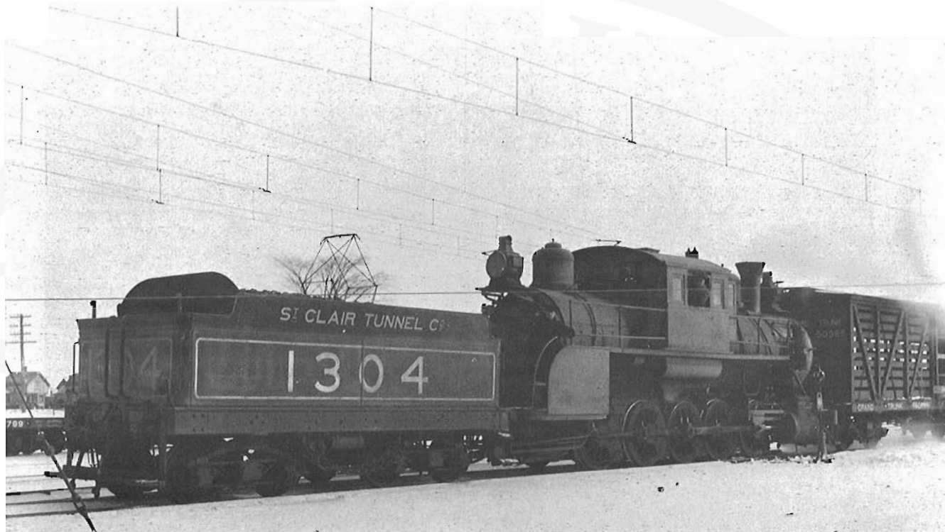
The modification of the tunnel locomotives from tank to tender equipped locomotives did not improve their aesthetics. This view, which was taken in 1908, shows the large firebox which challenged the fireman. Originally numbered 598 to 601, the quartet of tunnel locomotives were renumbered 1301 to 1304 in 1898. These units remained in yard service after being displaced from tunnel service. The first unit was retired in 1916 and the other three in 1920.
