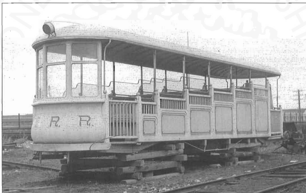
Edmonton Radial Railway observation car body is stored on blocks at the east side of the Cromdale Shop in 1945. Note the screening above the railings and the decorative wood panelling. Photograph by Bob Walker.
