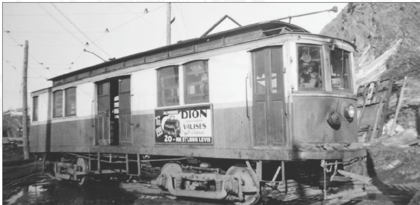
This freight motor was built by the Laconia Car Co. in 1903 and acquired by the Lévis Electric Railway for freight operation on the company's lines. This car survived the 1921 fire and was converted to a passenger car in 1942 and lasted until the end of service in 1946. Library & Archives Canada E008299366 Author's Collection
