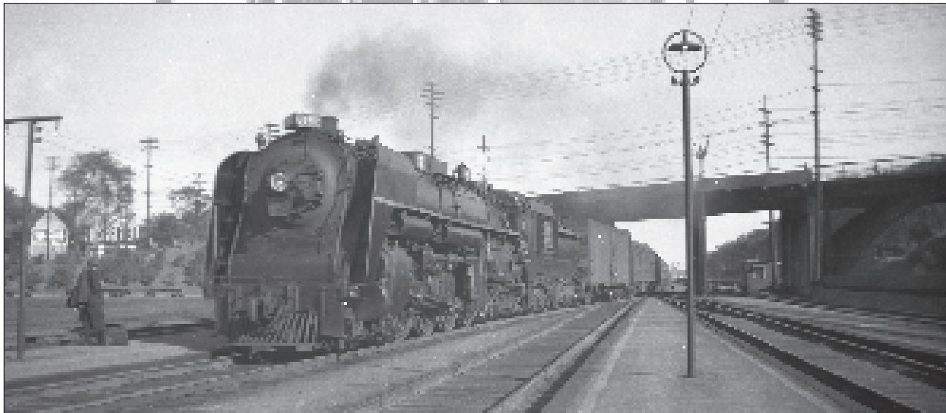
CNR U-2-h Northern 6252, a MLW 1943 product wheels Montreal-Ottawa train 51 under the Laurier Avenue bridge moments before bringing its train to a halt at the bumper post on a stub track inside the train shed. It's 6:55 on a weekday afternoon, circa 1950. The switch-tender's shack is visible just beyond the bridge alongside two double-slip switches at the throat of the station tracks. Addy Schwalm, Bill Linley collection.
