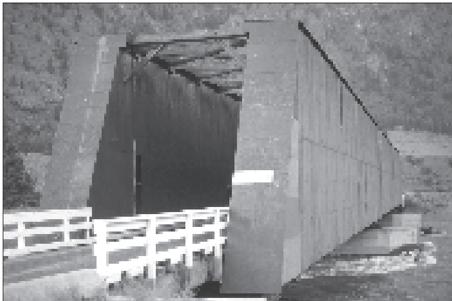
The wooden truss bridge just north of Keremeos survived the floods of 1972, it received concrete piers replacing the wooden ones. This view is from 1991, the bridge carries the Asnola road, access to the Cathedral Lakes Provincial Parks. Philip Mason.
