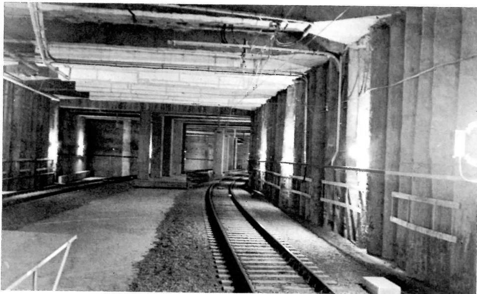
The downtown tunnel section looking inbound from Churchill Station. The walls consist of the bare underpinning columns. Note ties and ballast.
