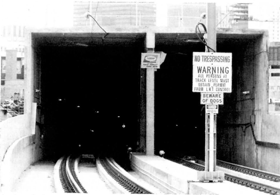
A view of the portal at 95 Street. The tracks at this point are bolted to a raised concrete guideway. The tunnels are patrolled by dogs at night.
