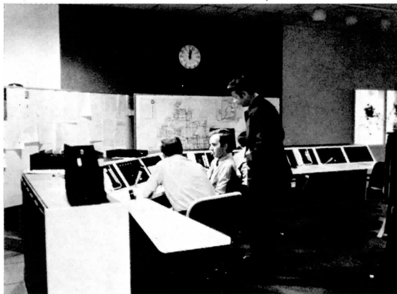
TOP LEFT: In the Transit Control Centre all stations can be monitored simultaneously by way of these television screens.
