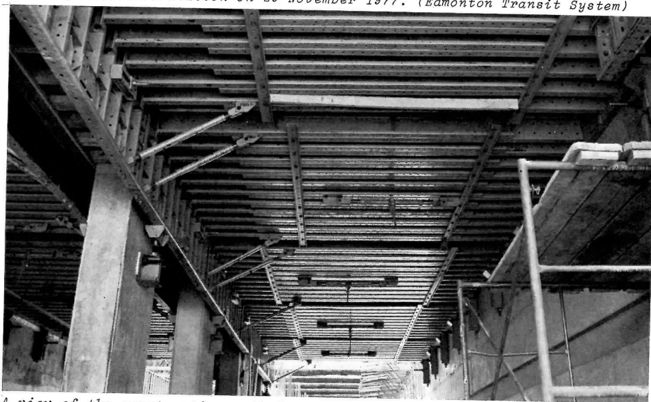
A view of the construction method used to build the roof/ceiling of the short tunnel south of Belvedere, 26 April 1977. (Edmonton Transit System)
