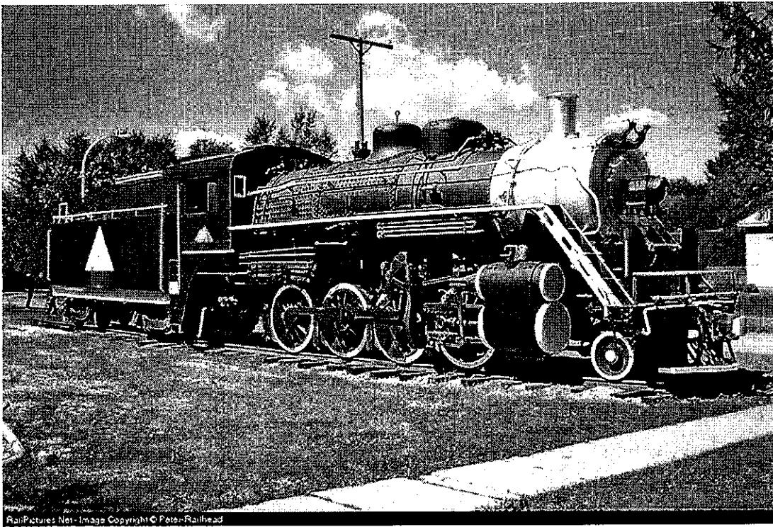
17 survived dieselization and later operated hauling freight and tourist trains on the Crab Orchard & Egyptian in the US for a few years before again being retired. During which time it lost its stoker, vestibule cab, feedwater heater, and superheating. It is on display in Boone, Iowa, September 6-2004.
