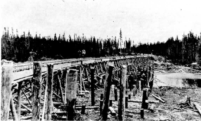
Dist. C. Res. B. Coffee River. Temporary & Permanent trestles Sep 27, 1912
