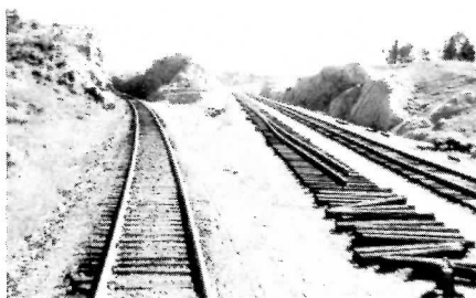
ABOVE CENTRE - The new grade has just been opened and the rails removed from the old grade as another section of double track route nears completion. (R.W. Layton)
