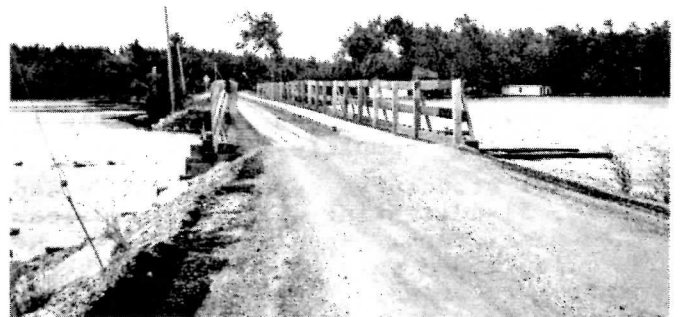
Looking across the former C.P.R. wooden trestle over the Otonabee River. The bridge has been converted for "single track" automobile use by the addition of longitudinal planking strips and wooden side railings.
