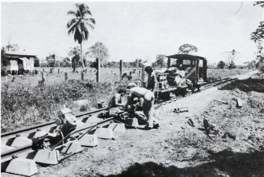
Track laying, Costa Rica style: a joint crew comprising natives and CP Consulting Services personnel is busily joining rail sections on the 65 mile line which has been undergoing rehabilitation. The corkscrew-like metal clips fastening the rails to the concrete ties are similar to those used in the open cut sections of the TTC's Spadina Subway. CP Rail photo
