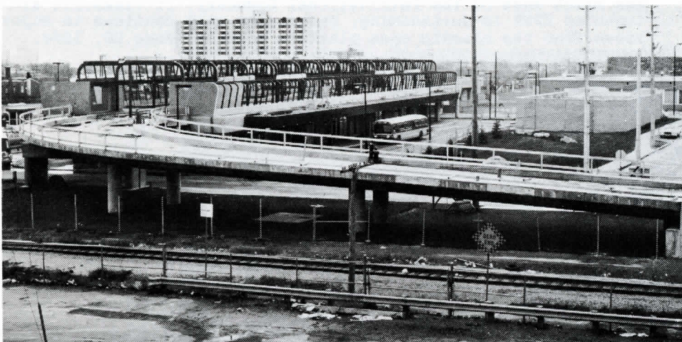
The TTC's Kennedy Terminal, shortly after opening, looking southwest from the Eglinton Ave. overpass. The SLRT ramp is completed except for parapets; work has begun on the LRT platform walls, while material for covering in the roof awaits installation. CNR Uxbridge Sub. in foreground, pedestrian entrance and substation structure behind ramp.
